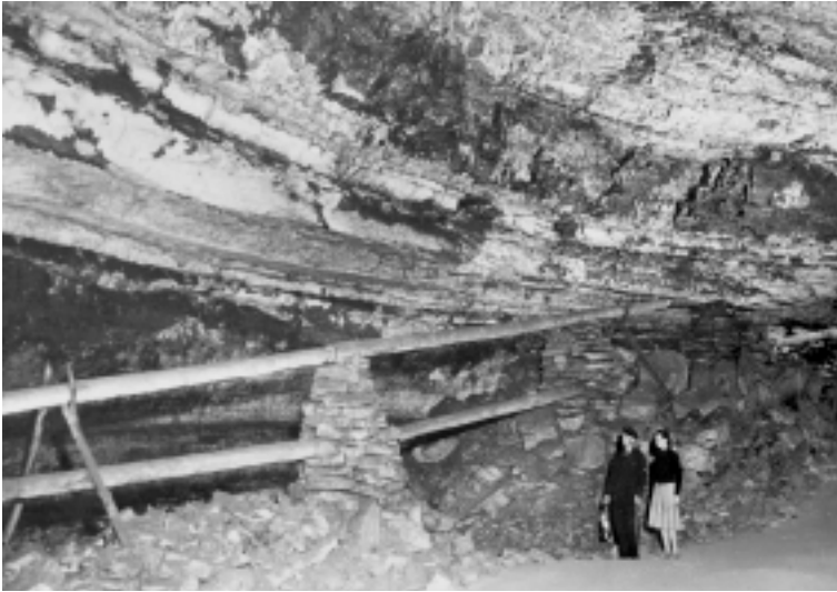
Figure 2. Remains of the Mammoth Cave saltpeter works. Pipes carried water from a stream at the cave entrance to leaching vats where the saltpeter was recovered. Undated photo courtesy of the Kentucky Library, Western Kentucky University.
